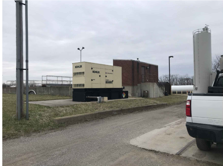
DIESEL GENERATOR (300 KW) NO SCALE
