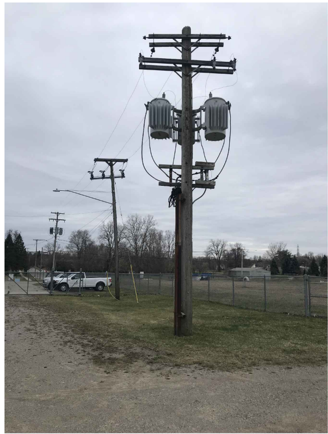
SOUTH ELECTRICAL SERVICE POLE-MOUNTED SWITCHES, TRANSFORMERS, AND METERING NO SCALE
