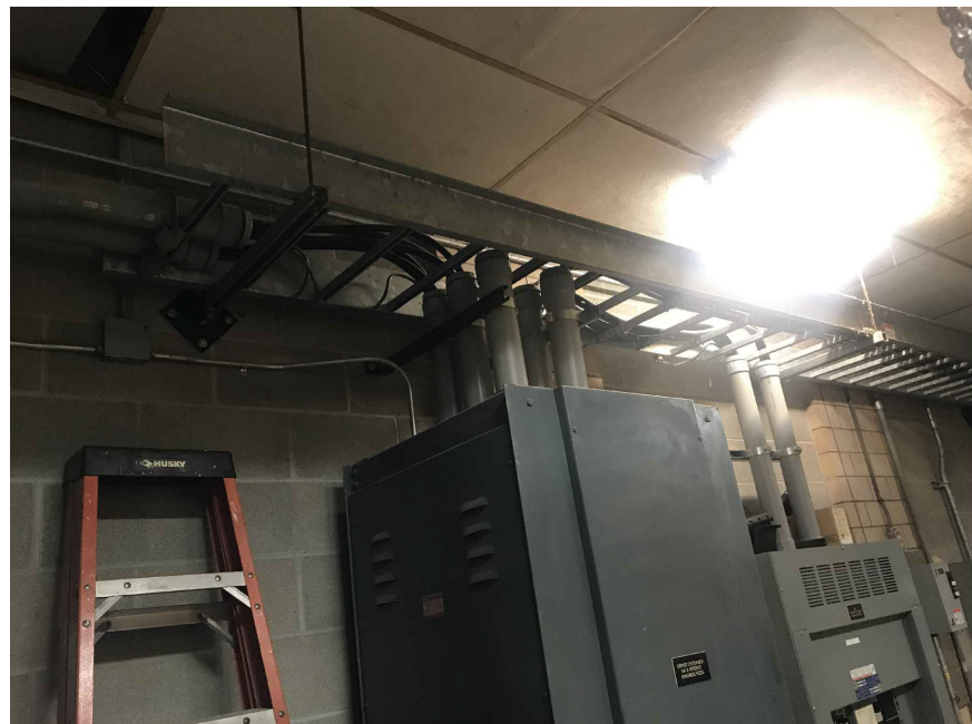
ELECTRICAL ROOM CABLE TRAY NO SCALE
